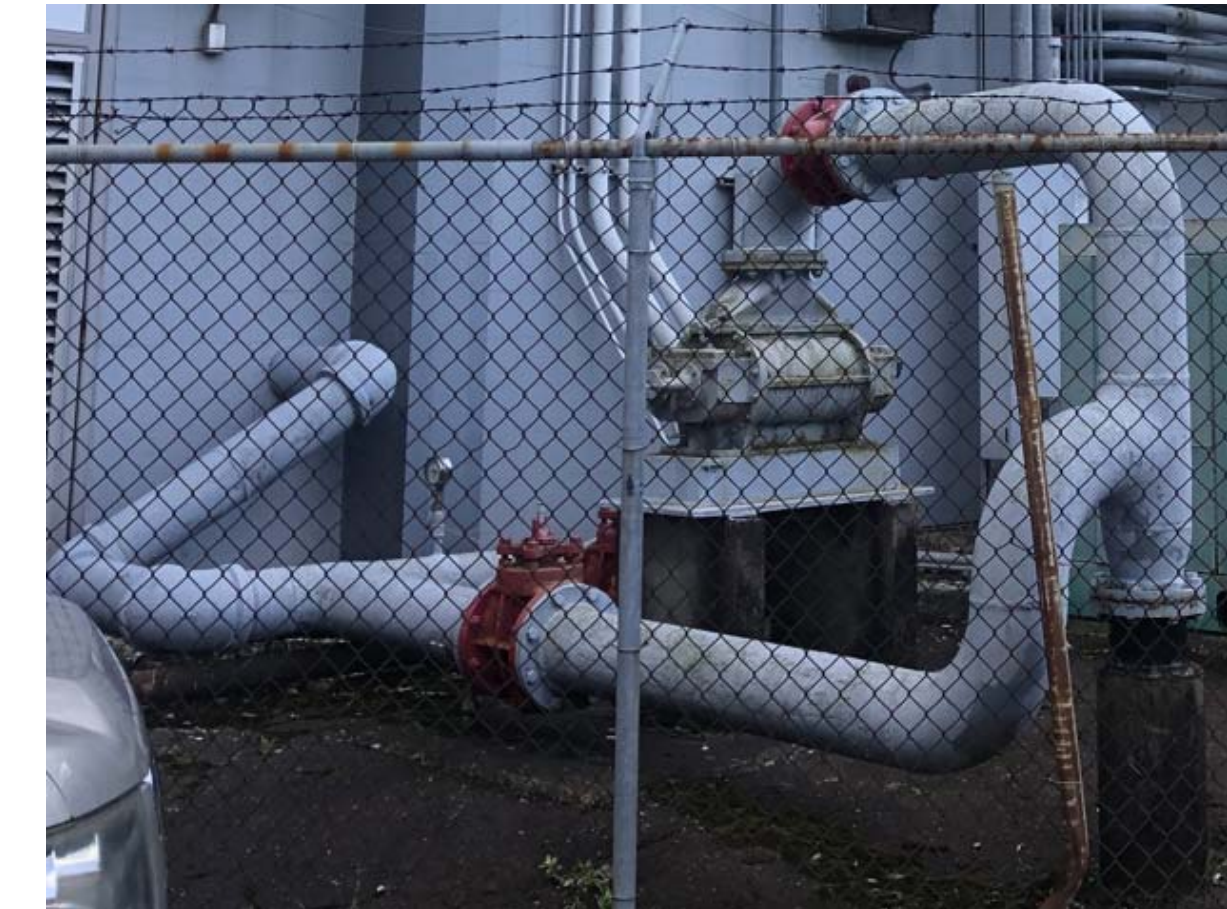
② EXISTING INCOMING GAS MAIN SCALE: 1/4" = 1'-0"
