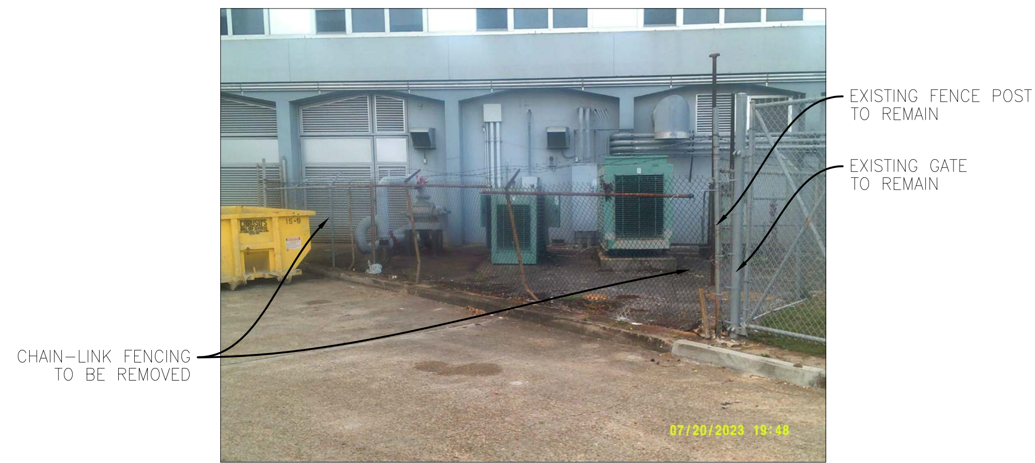
P1 EXISTING FENCING VIEW
