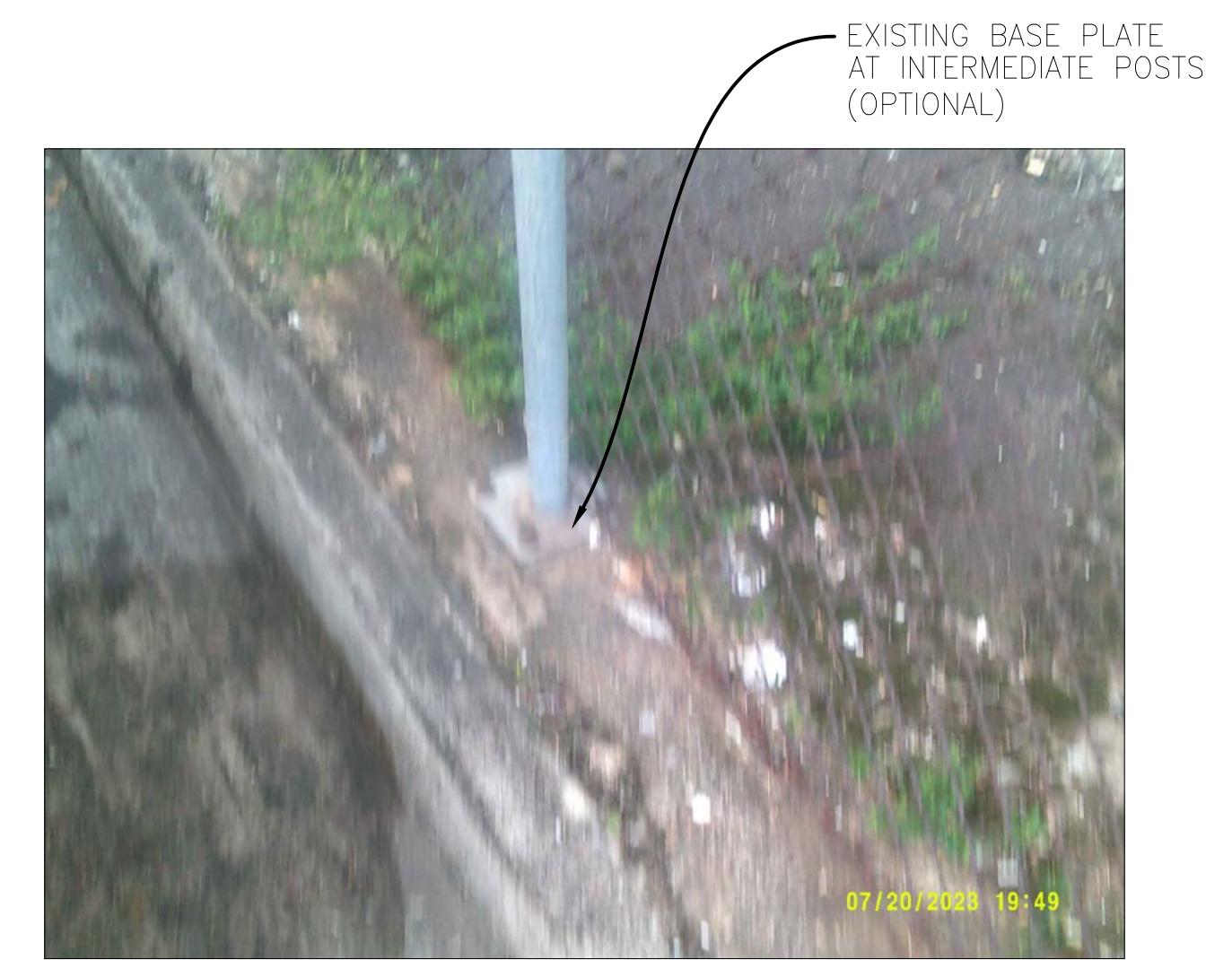
P2 BASE PLATE AT FENCING
